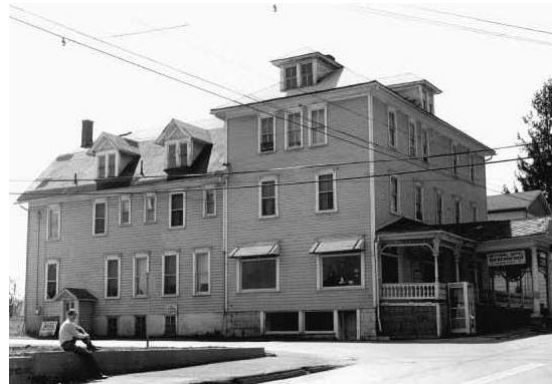
The many historic sites and structures associated with the Old National Road in Garrett County are an important historical legacy for the nation.
