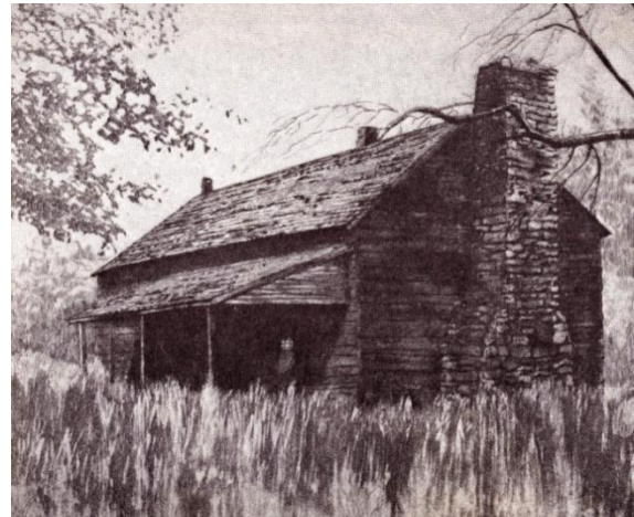
The James Drane House in Accident Maryland is one of the County's oldest remaining structures (circa 1800).
