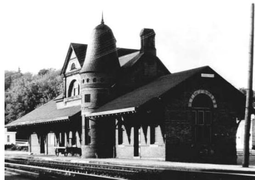
The B&O Railroad in Oakland is one of the County's most significant historic sites and structures. It was recently deeded by the Town to the Garrett County Historical Society for management.
